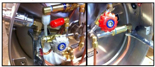
3. Use a 5/64" Allen socket and 7/16" box end wrench, loosen and remove the fill receptacle mounting bolts. Retain the mounting bolts and fill receptacle protective cap for re-use.
