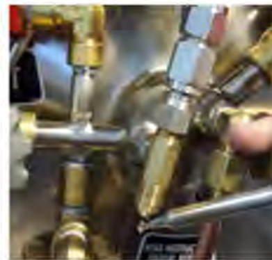
DIRECTLY FROM TANK CAPACITANCE WIRE – FEED THROUGH DISCONNECTED
