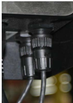
Fig. 6 - Temp Probe Installation on TEC3000
