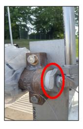
We do recommend that these parts be replaced as soon as convenient. Chart will provide replacement B16.11 parts, which are properly rated. The part number for the proper fitting is 11803562.
