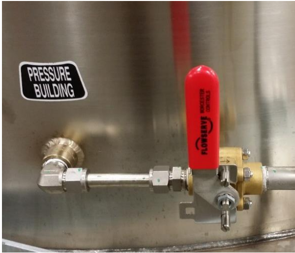
Old Style short stem cryogenic Worcester Valve. p/n 1712202
