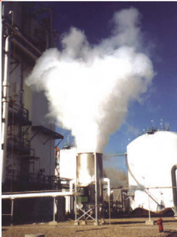
Thermax FAD 250 on 55,000 lb/Hr O 2 N 2 capacity at exit temperature 50°F below air temperature
