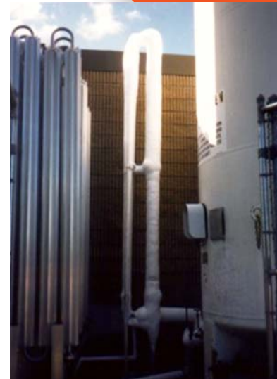
Two Ice Racks Model IR-9, Two Super-Gap Ambient Vaporizers Model TF3618HF•SG
