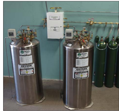
A typical Chart Perma-Cyl Medical Oxygen System
