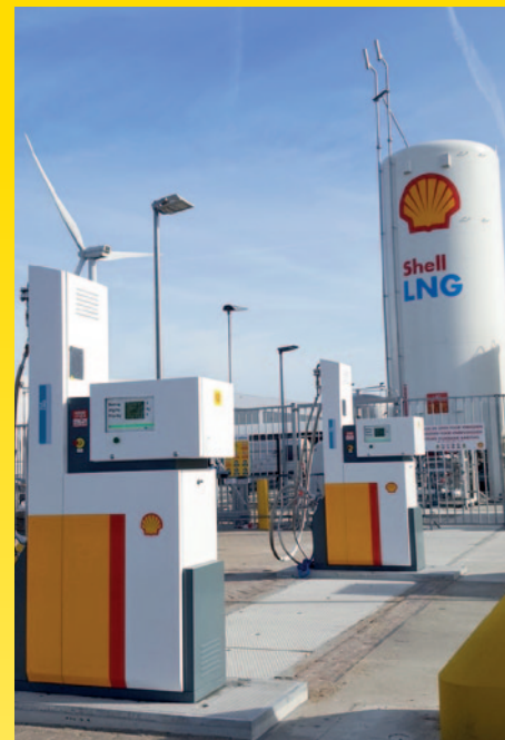
Stanice pro firmu Shell, Rotterdam
