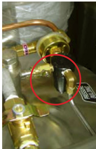
Figure 3: Pressure Builder valve and Vibra-Lok fitting (Carbo-Mite, Charger, Mizer)
