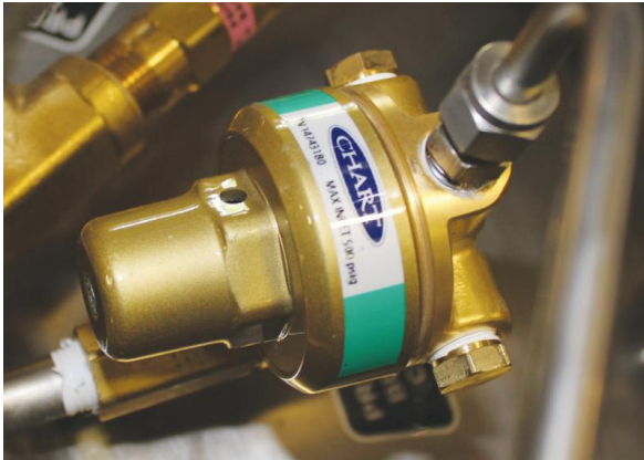
Pressure building regulator on a Carbo-Mizer ® style tank.
