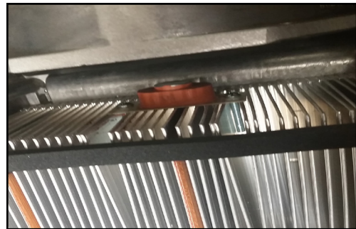
Figure 9 - VFD Thermostat Installed
