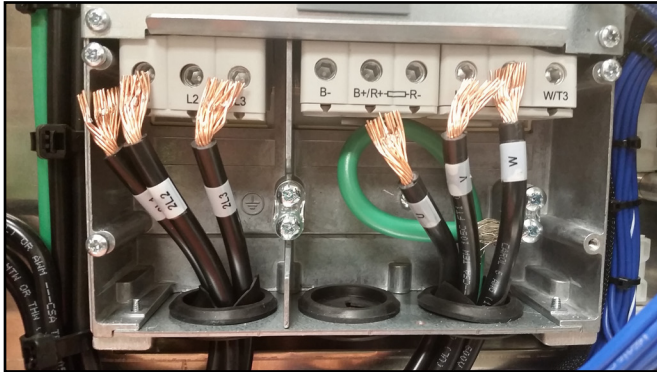
Figure 6 - Front cover removed for access to wiring.
