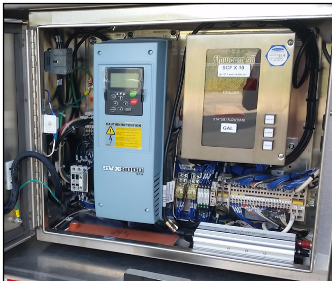
Figure 4 - Control Panel with 110V Heater System
