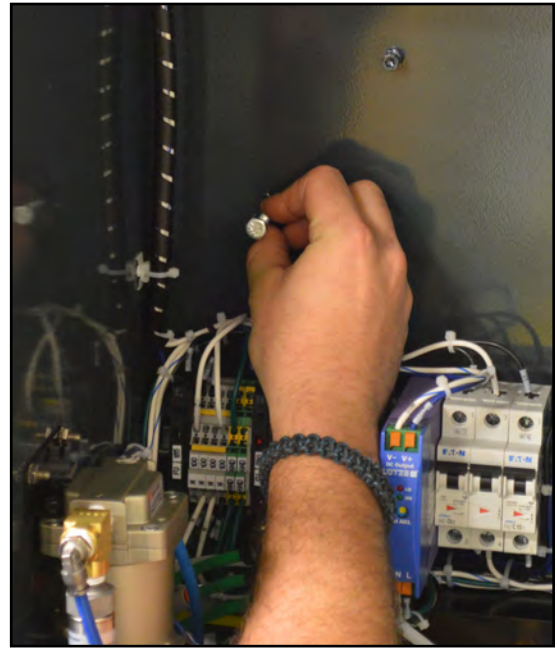
Photo 5 - Installing the safety lock screw into the cabinet.
