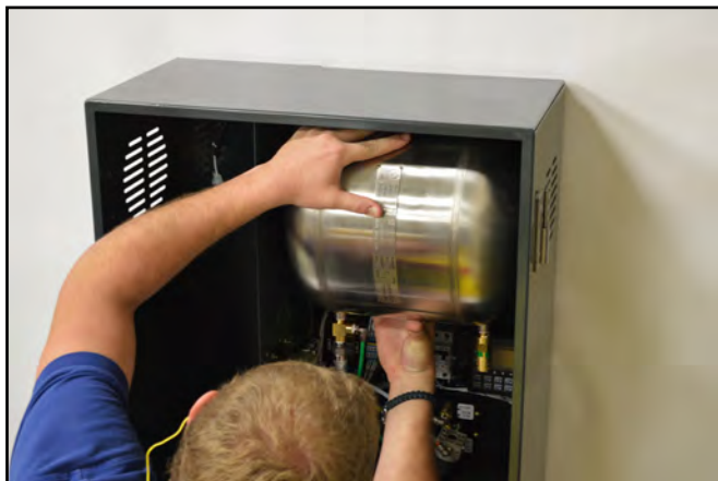
Photo 7 - Installing the stainless steel N 2 tank
