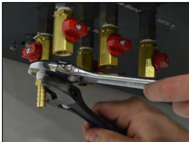
Photo 22 - Proper use of backup wrench
