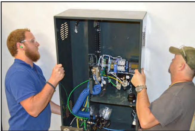
Photo 4 - Sliding the cabinet onto the mounting bracket
