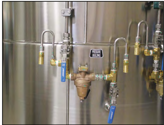
Figure 4 - PB Regulator with Isolation Valves
