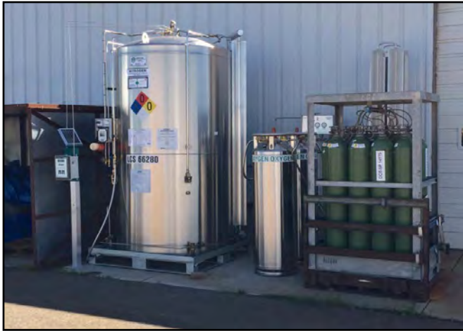
Perma-Cyl 2000HP with external pressure build vaporizer
