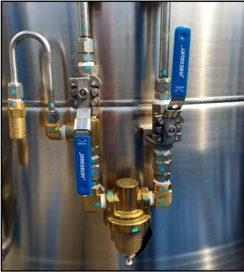
Figure 6 - Economizer Regulator with Isolation Valves
