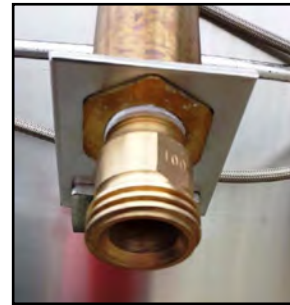
Figure 1D - 1" CGA Fitting shipped on Perma-Cyl CO 2 2000/3000 HP tanks
