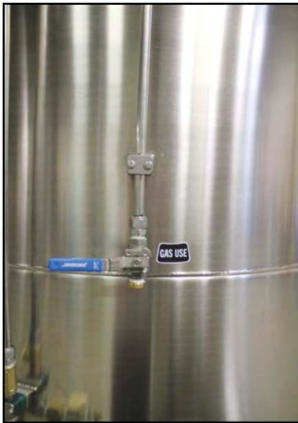
Figure 8 - Gas Use ball valve
