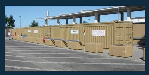
Chart's IMC-6000 fuel station is self-contained, preassembled and tested. The system is mounted inside a standard 40-foot ISO container and provides the following advantages:
