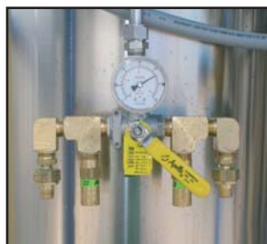
Dual Relief Valve Assembly
