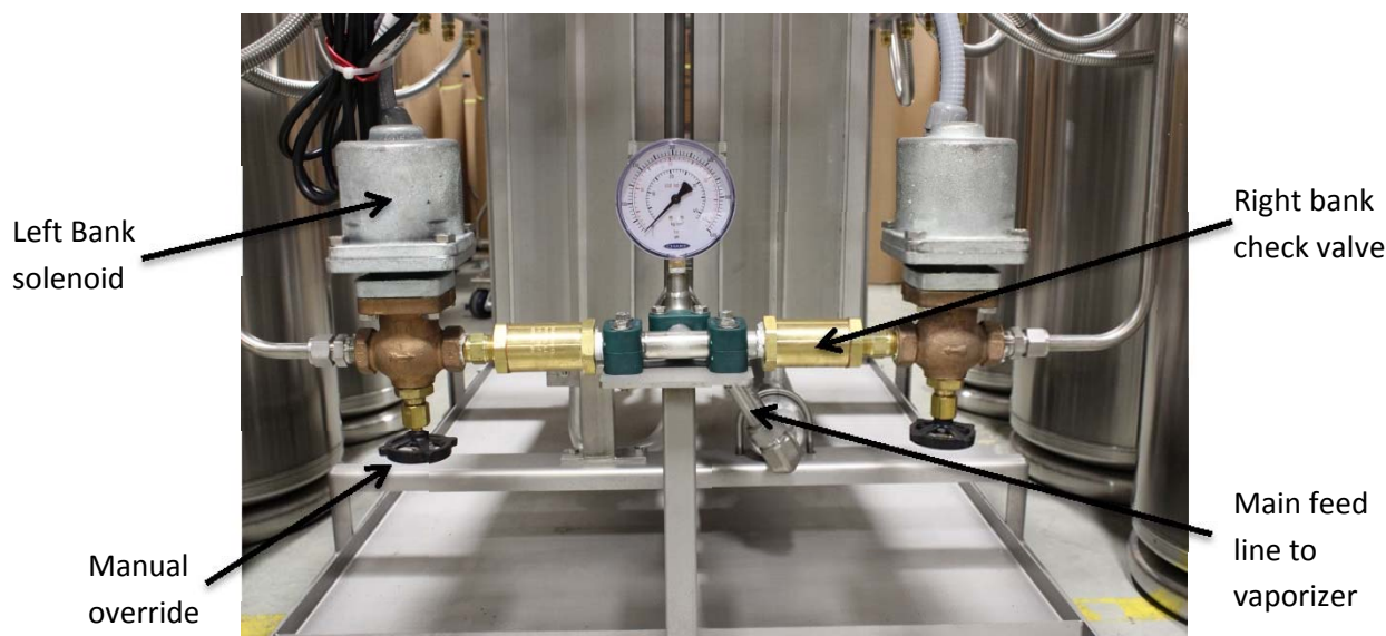
Figure 6: Solenoids, check valves, and main feed line to vaporizer
