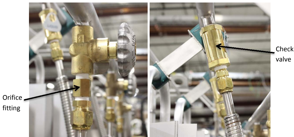
Figure 5: Orifice on lower (vent) header and check valve on upper (liquid) header
