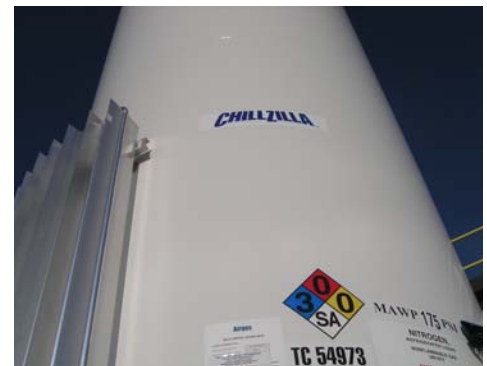
ChillZilla® 11,000 gal. with high flow 40 gpm vaporizer and 2" VIP withdrawal
