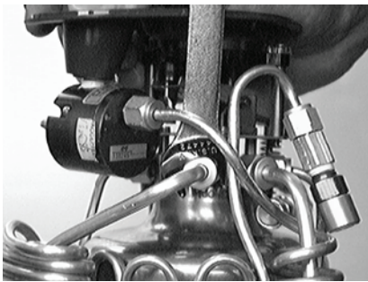
Figure 17: Warming Coil Removal
