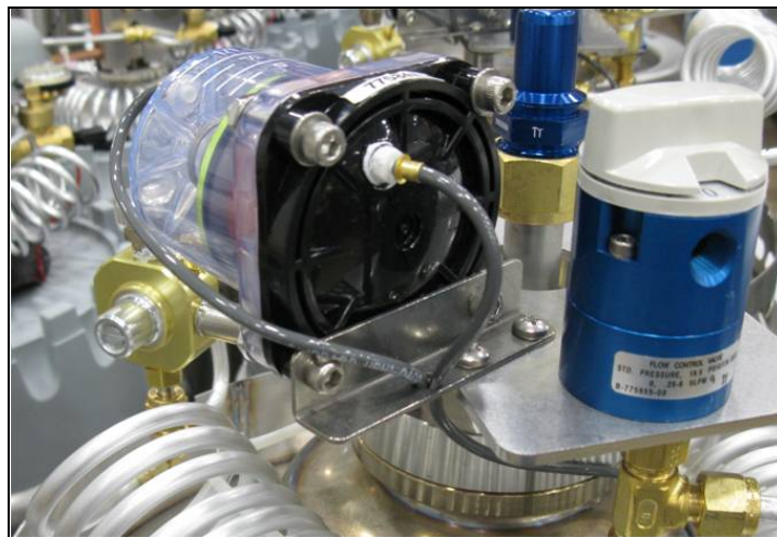
Figure 2 - - Old LLG Sensing Line Routing
