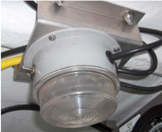
Service Lights Switch (Interior Cabinet)
