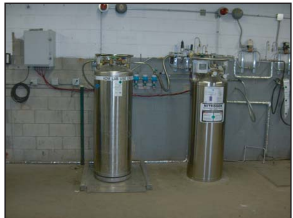
Lo-Loss & Argon Maximizer Installation
