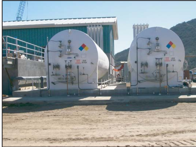
System installation at site (Note vaporizers in background.)
