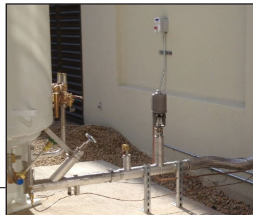
E-Stop control system with integrated actuated valve
