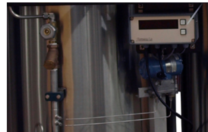
Differential Pressure Flow Sensor
