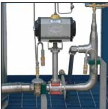
Automatic Fill and Safety Shut-Down Valve
