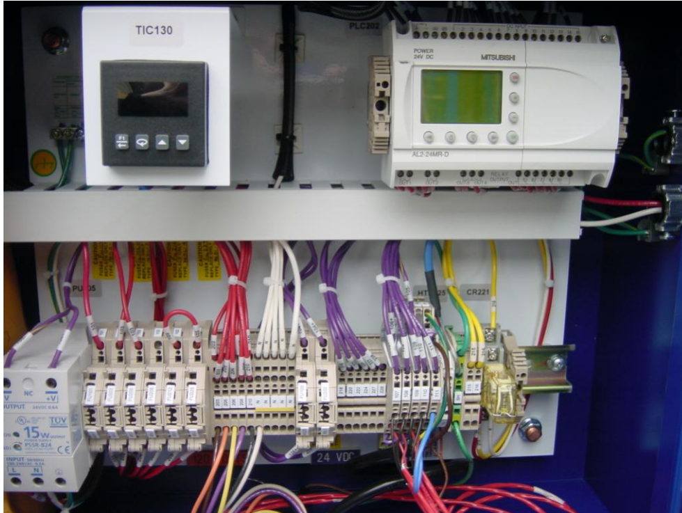
Figure 9 - Trifecta X-Series Control Box (open)
