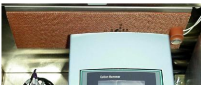
Control Panel Heater
