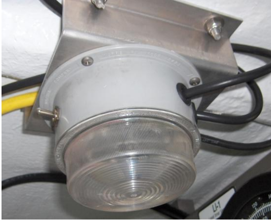
Service Lights Switch (Interior Cabinet)
